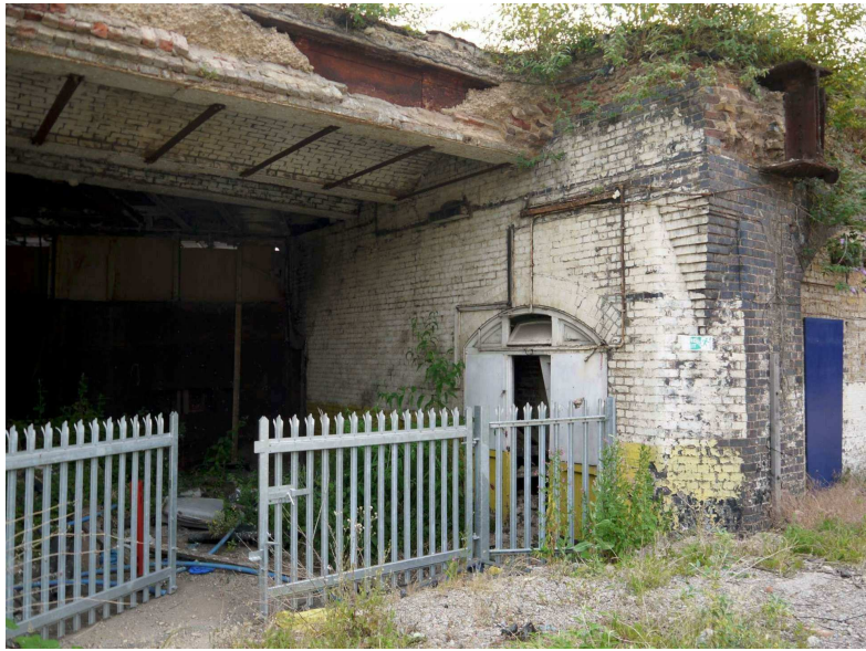
EXISTING EASTERN SIDE TO ORIEL GATEWAY - Partially collapsed lid & brickwork from previous demolition. Brickwork is irregular and unfinished. Fill material above arches lacks any retaining element to ensure stability of the remaining arches.
