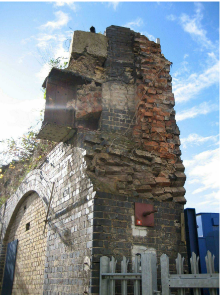
EXISTING NORTH EAST CORNER - Partially collapsed remnants of former arches from previous demolition for the London Overground. Fill material above arches lacks any retaining element to ensure stability of the remaining arches.
